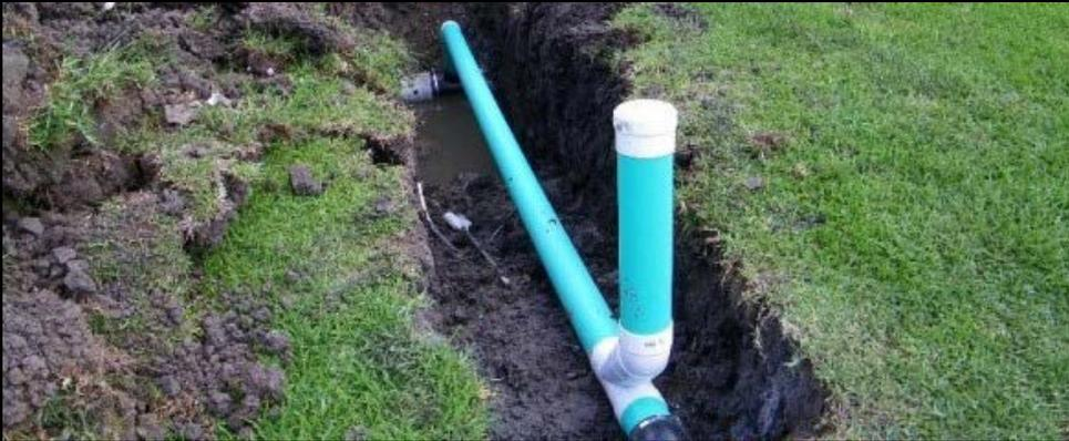
SEWER LATERAL CLEANOUT ALLOWS ACCESS TO LATERAL
