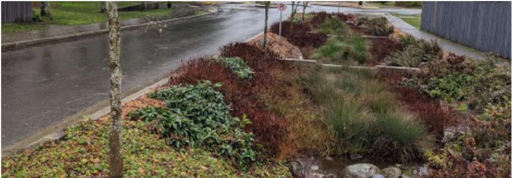
*Bioswale collects and filters stormwater
