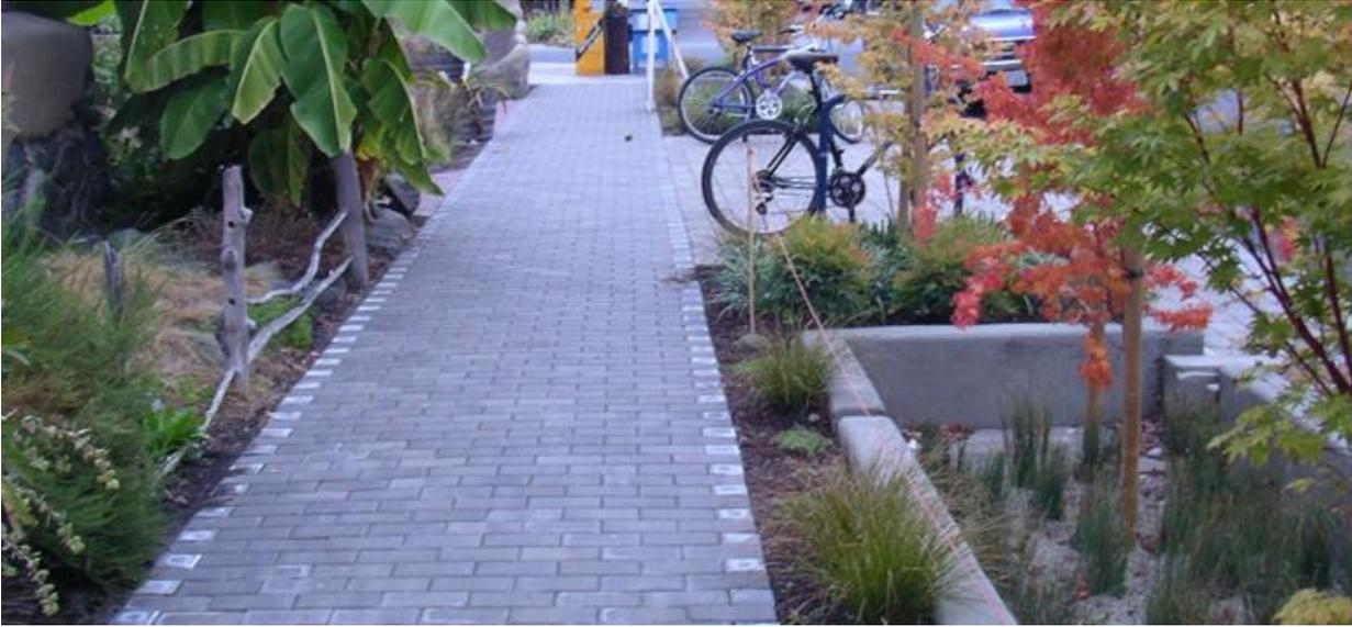
*Permeable paving and landscaping capture and percolate stormwater runoff
