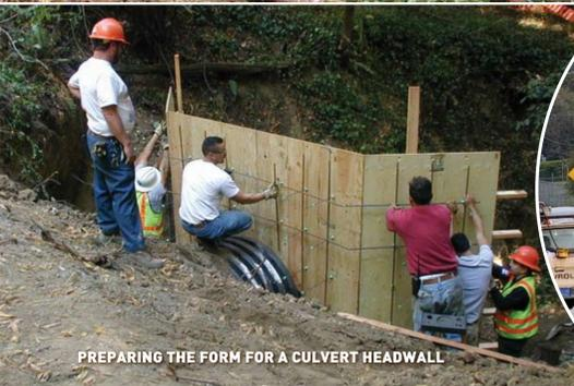
PREPARING THE FORM FOR A CULVERT HEADWALL
