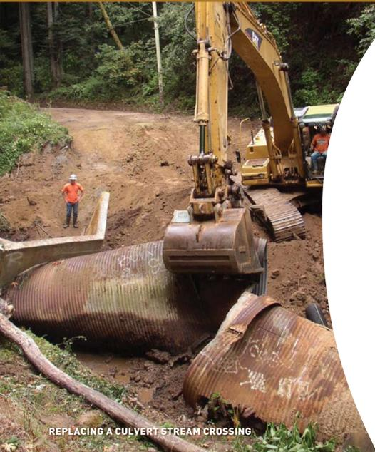
REPLACING A CULVERT STREAM CROSSING
