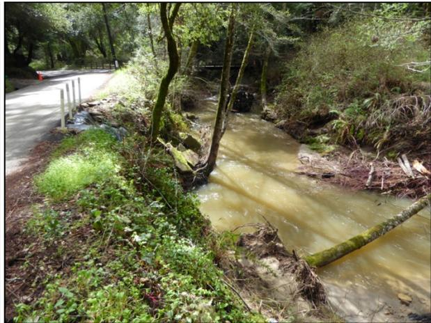
LEFT: Eroded left bank and scour pool at toe of slope.
