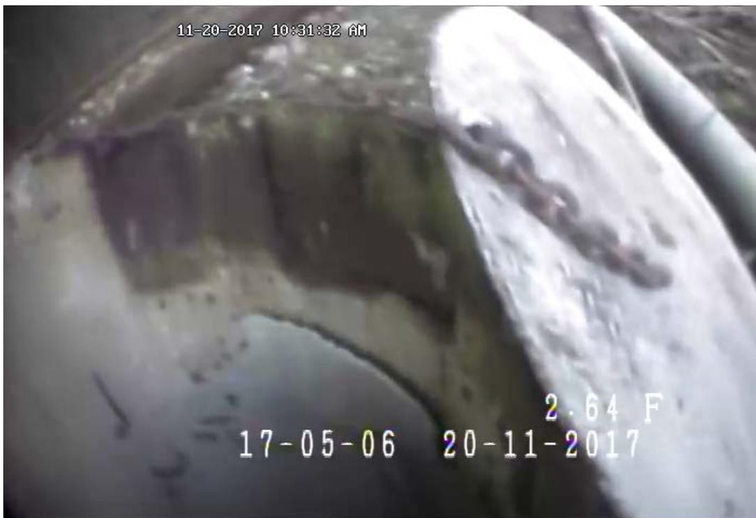
**Photograph 4:** Exterior view of the western shaft with lid at transition to Highway 1 culvert.
